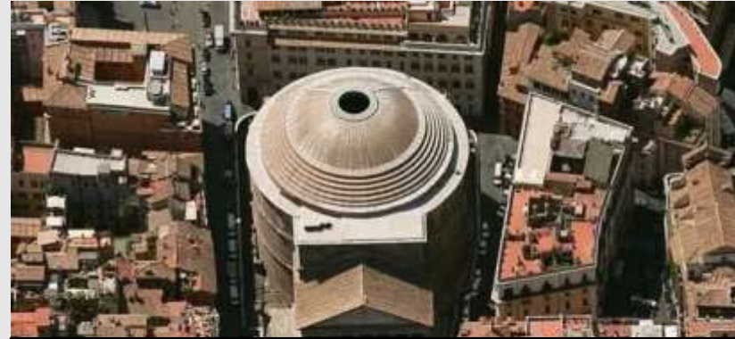
The Pantheon Dome (above) 43.4 m span 2,000 years old and still the world's largest concrete dome suspended without reinforcement.
